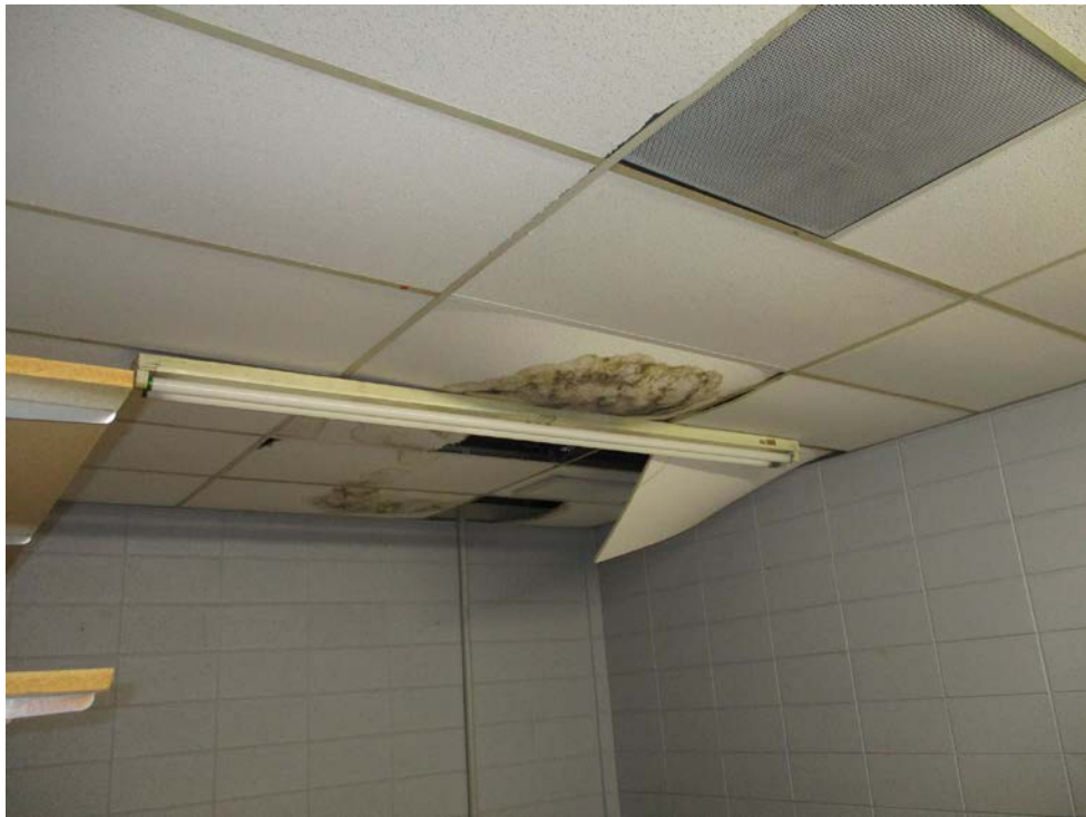
INTERIOR PHOTOGRAPH, WATER DAMAGE TO CEILING
