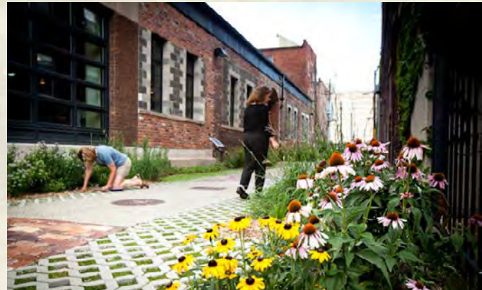
Permeable paving and bio-swales repurpose alleys into usable open space.
