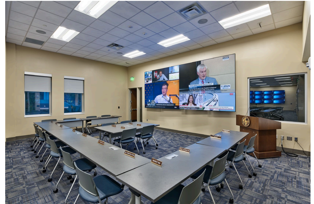
Example of current video wall technology at Emergency Operations Center
