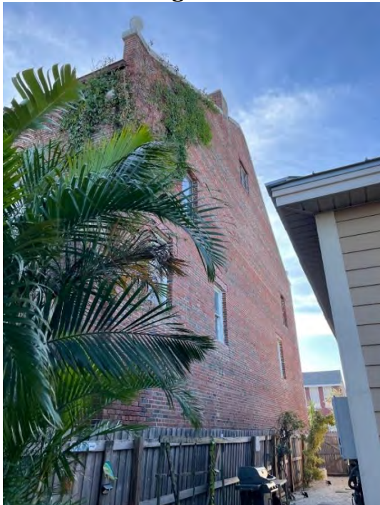
Figure 6 North Side Current Window Photo from Home
