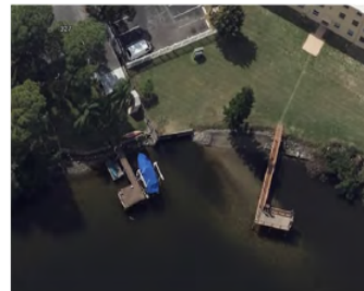
Existing 54" RCP outfall east of 87 th Ave N
