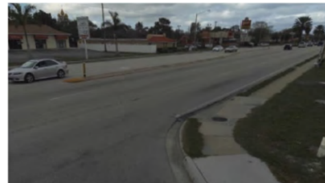
Existing intersection of 89 th Ave N & 4 th St N
