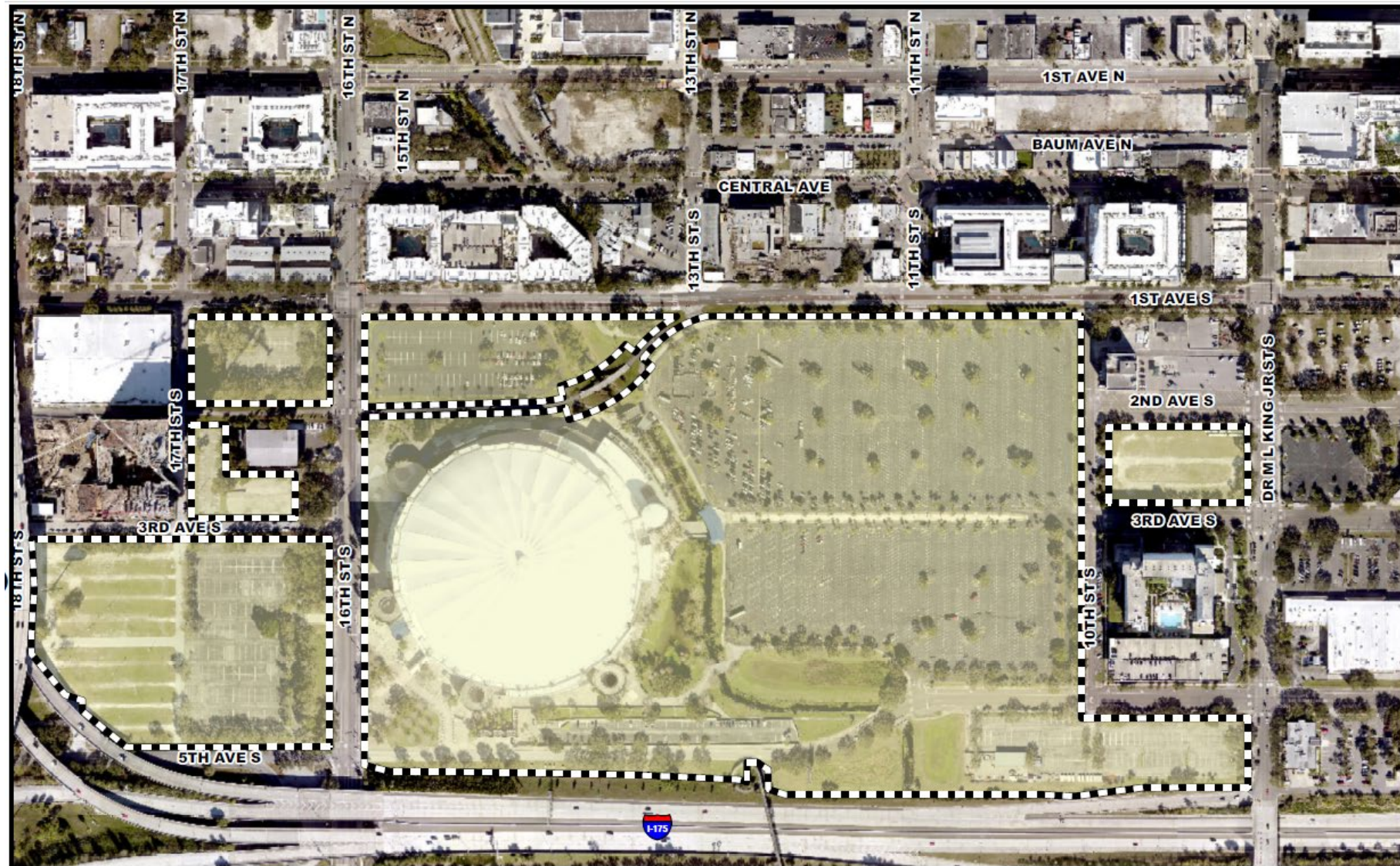
Historic Gas Plant District Development Agreement
