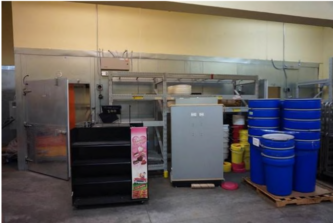
Interior of Building 1
