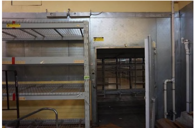
Interior of Building 1
