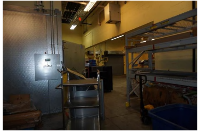
Interior of Building 1
