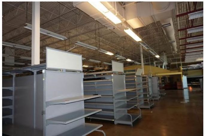
Interior of Building 1
