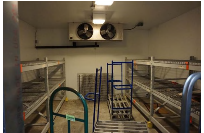
Interior of Building 1
