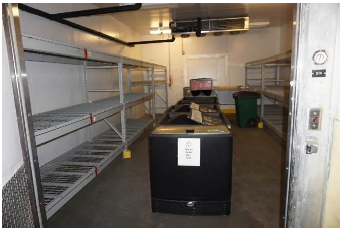
Interior of Building 1
