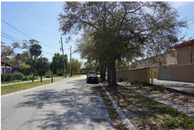
View Looking South Along 21 st St S (Subject on Right)
