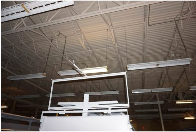
Interior of Building 1
