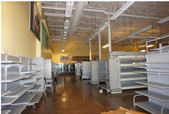
Interior of Building 1
