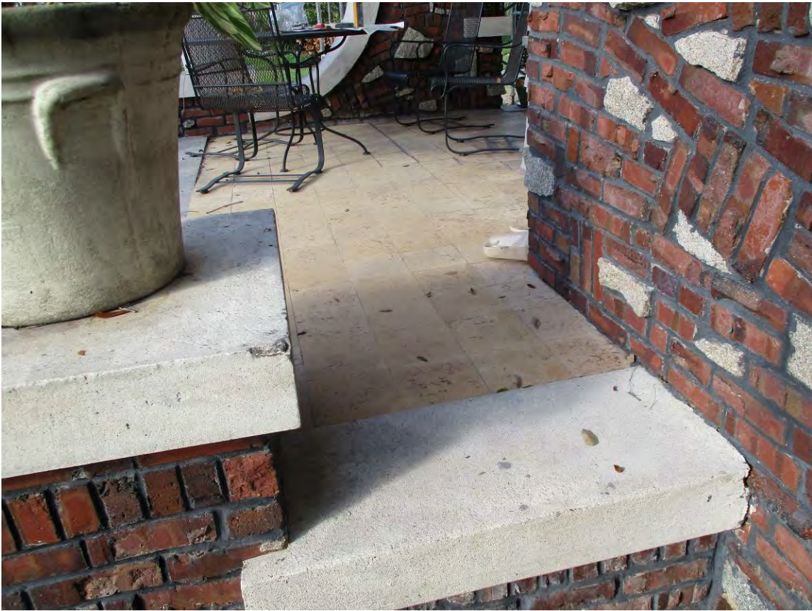
Photo 3: Frontal porch masonry with Cuban tile.
