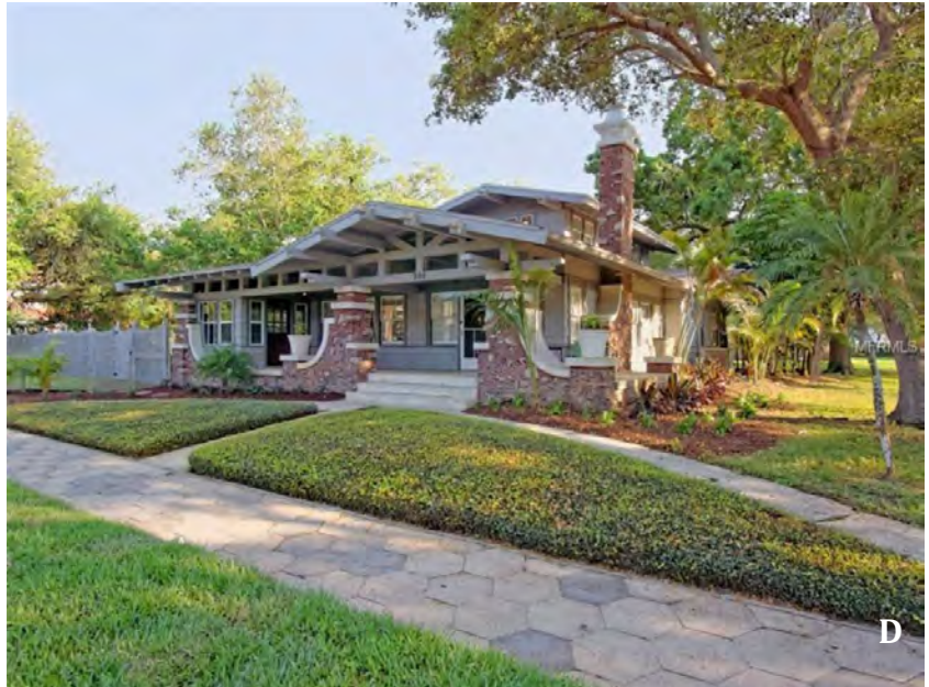
A. North facade Clinker brick pier
