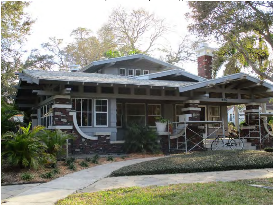
Photo 2: Frontal view showing gables and exposed eaves and truss system.
