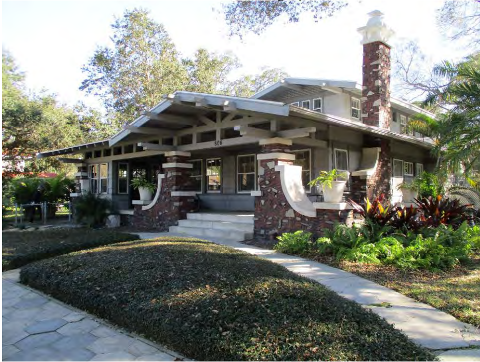
Photo 1: Oblique view of façade facing southeast.
