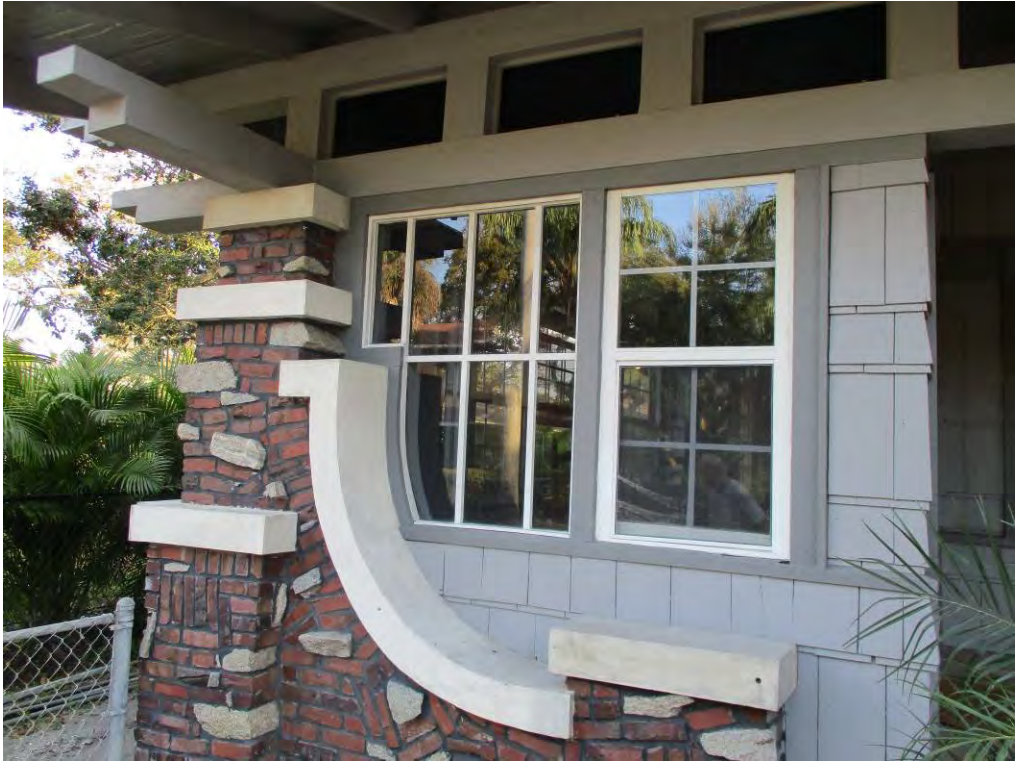
Photo 5: East porch enclosure at front elevation, with masonry workmanship.
