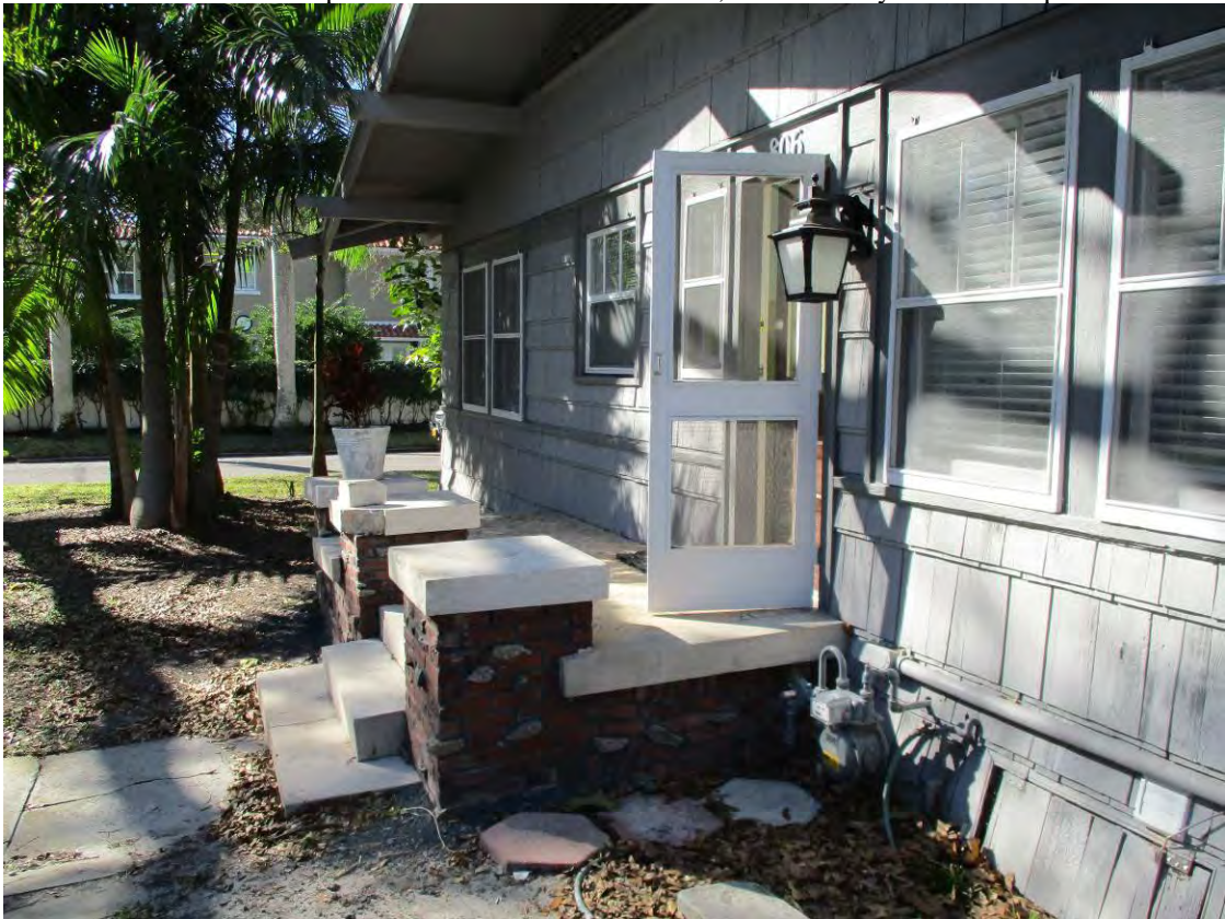
Photo 6: Rear porch area.
