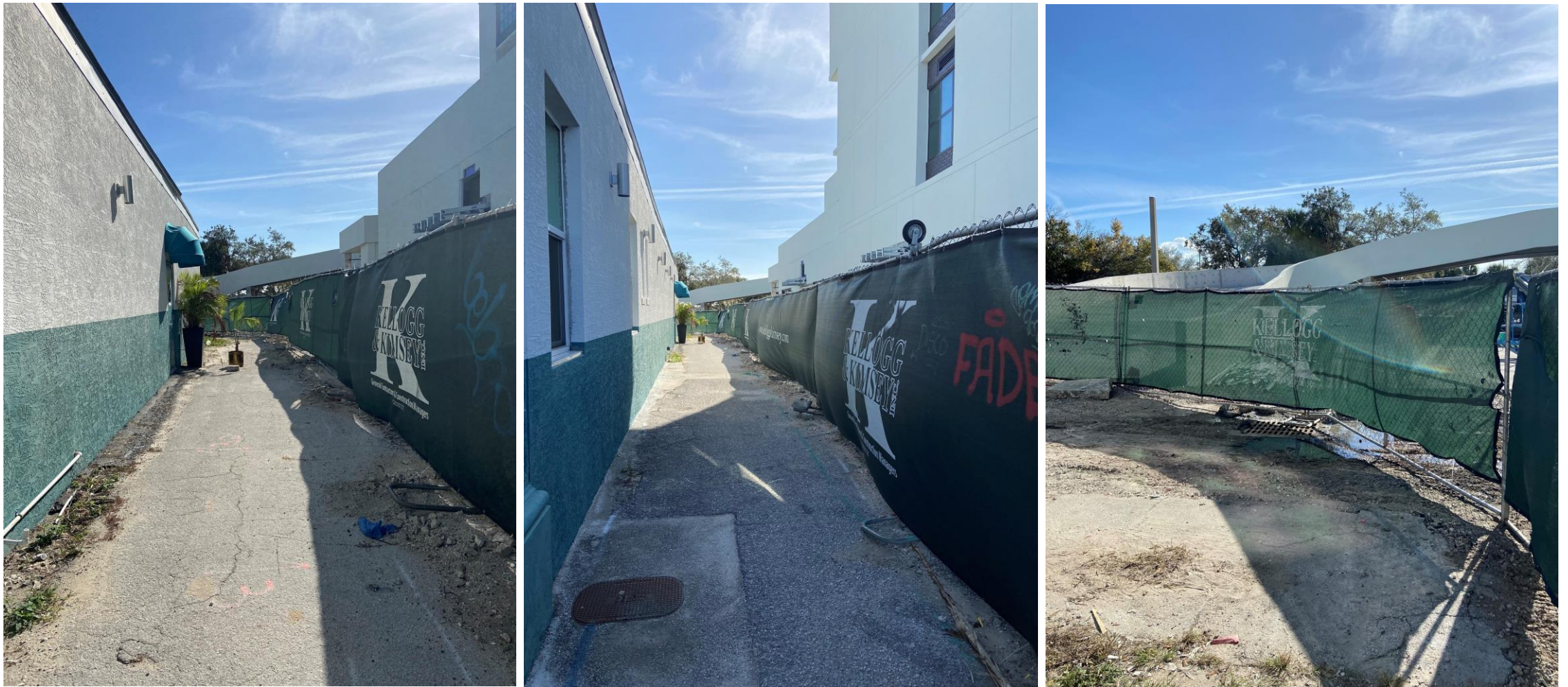
Southward view along the north-south alley to be vacated. Parking garage ramp to the Moxy project in the background.
