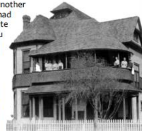
The Blocker House at 145 Fourth Ave. NE, Constructed in 1905 and photographed shortly thereafter
