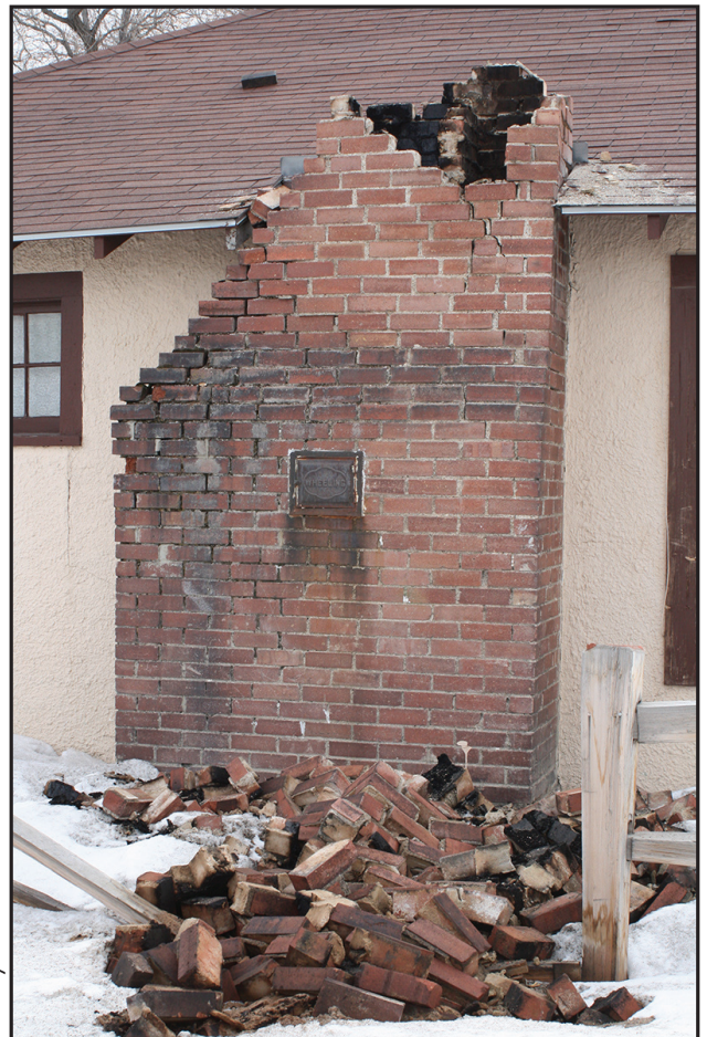
Damage to chimney from the 2008 Wells, Nevada earthquake. Everyone should be made aware that the areas around chimneys are dangerous during earthquakes.
