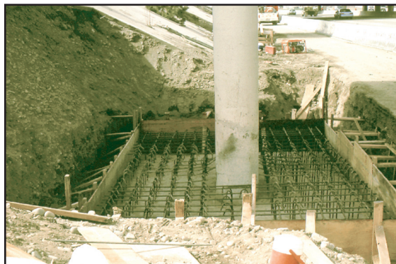
Seismic strengthening of bridges in western Nevada.
