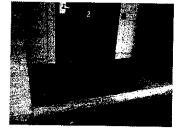
4. **Issue:** Side entrance: approach has sections with running slope >5%; door lacks minimum 48" wide clear maneuvering space for latch pull-side approach.
