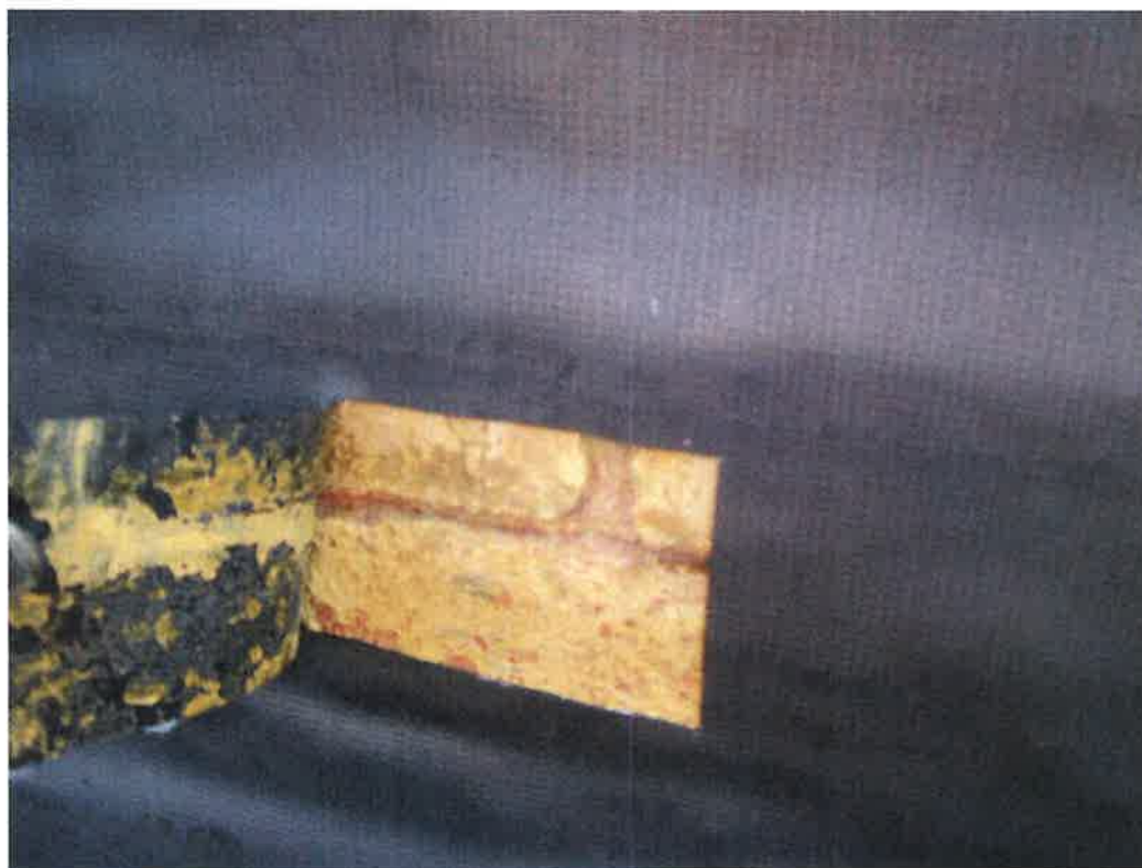
Parapet wall and membrane adhesive (1937 Section)
