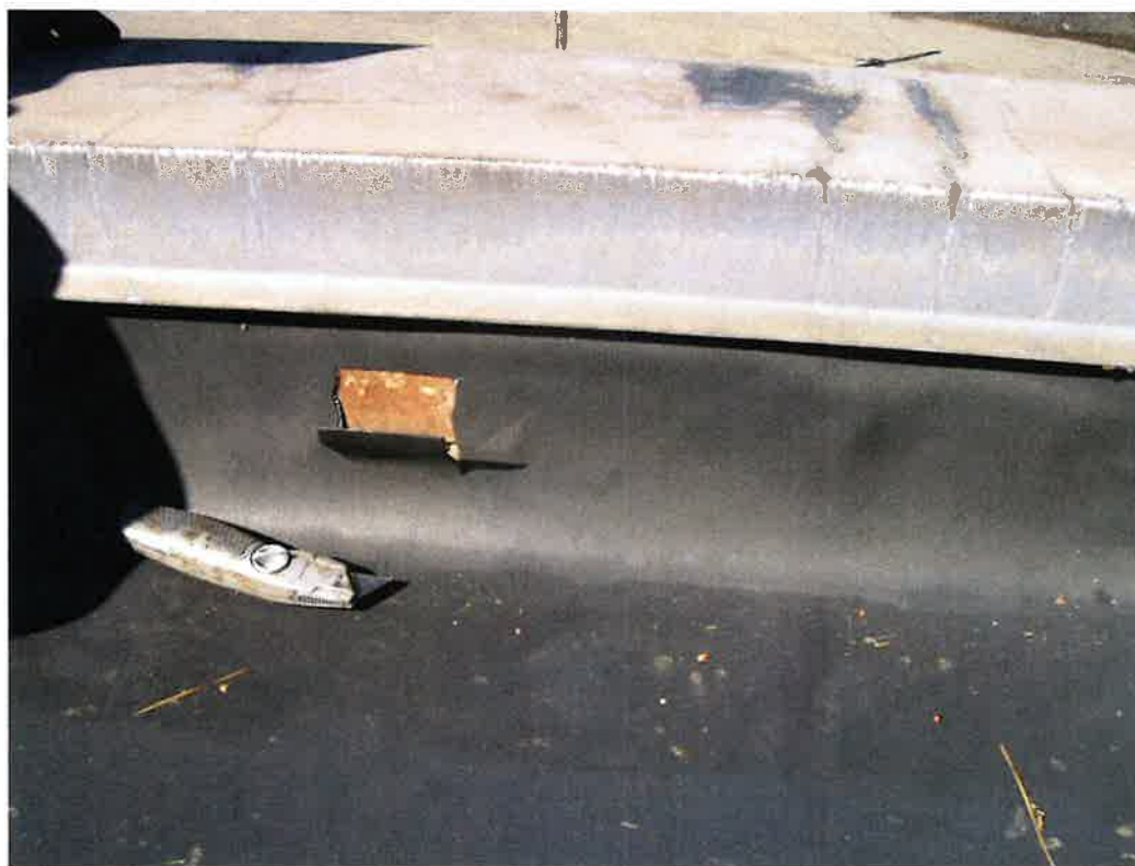
Low roof parapet wall adjacent to Gym (West side) – exposed brick behind membrane
