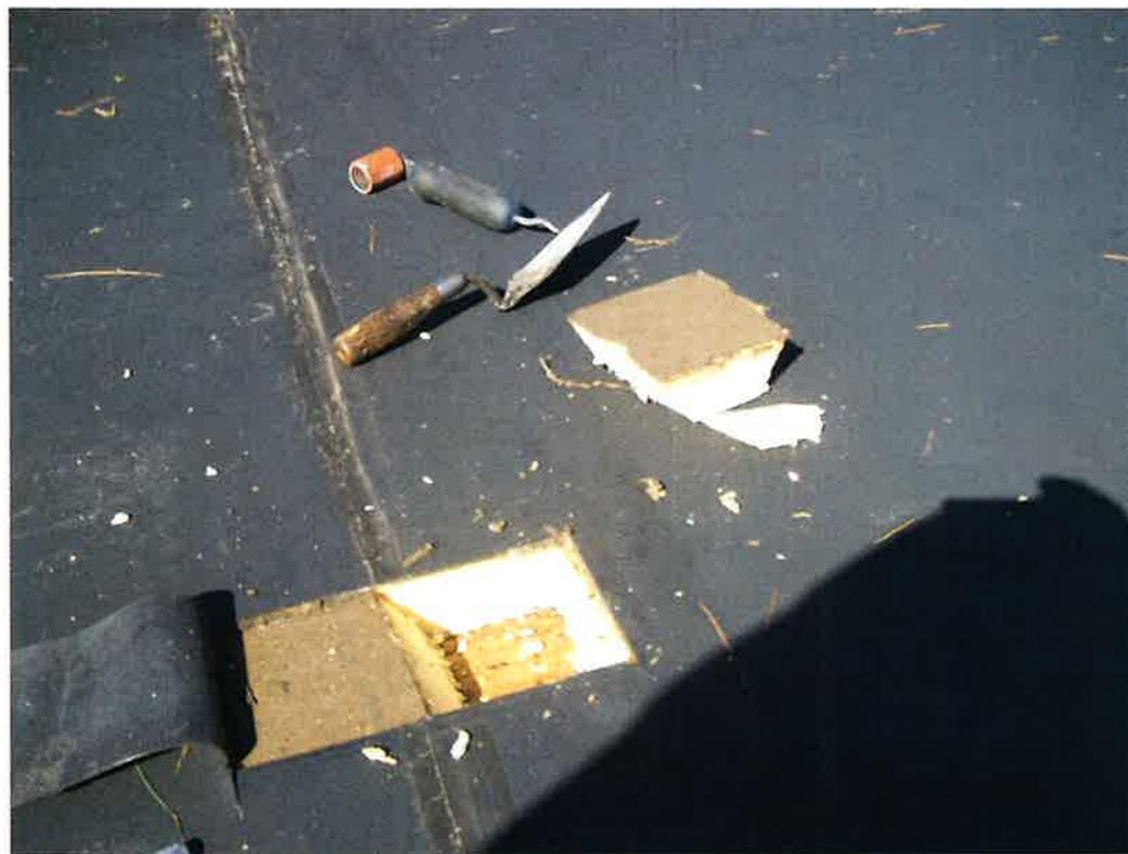
Gym Roof layers-wood decking exposed
