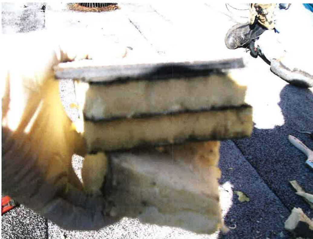
1991 Addition, low roof-layers of built up roof
