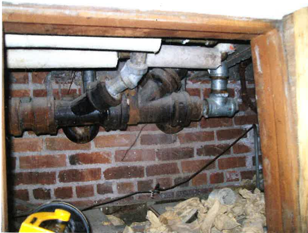
Pipe ACM inside wall cavity of first floor boy's room-hatchway entrance
