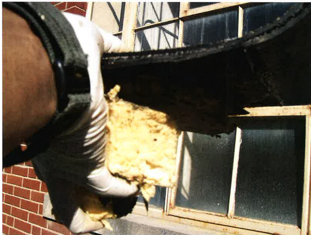
1991 Addition, low roof-back edge, layers of built up roof
