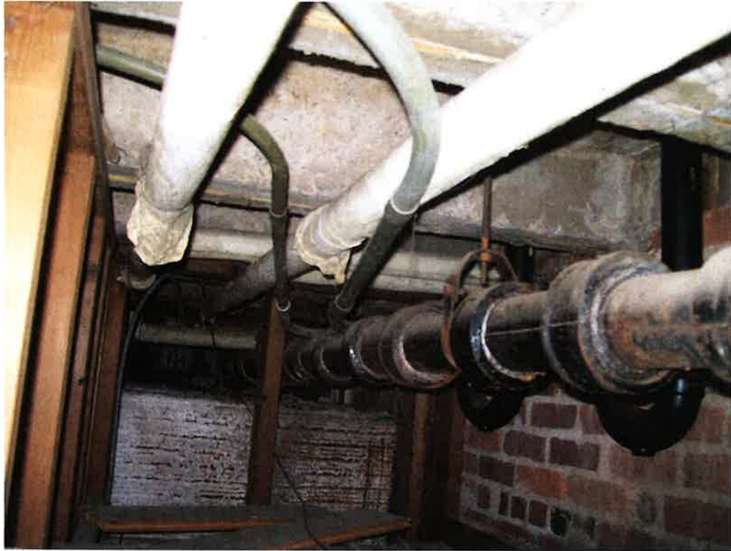
Pipe ACM inside wall cavity (as seen from 1 st floor boys' room)
