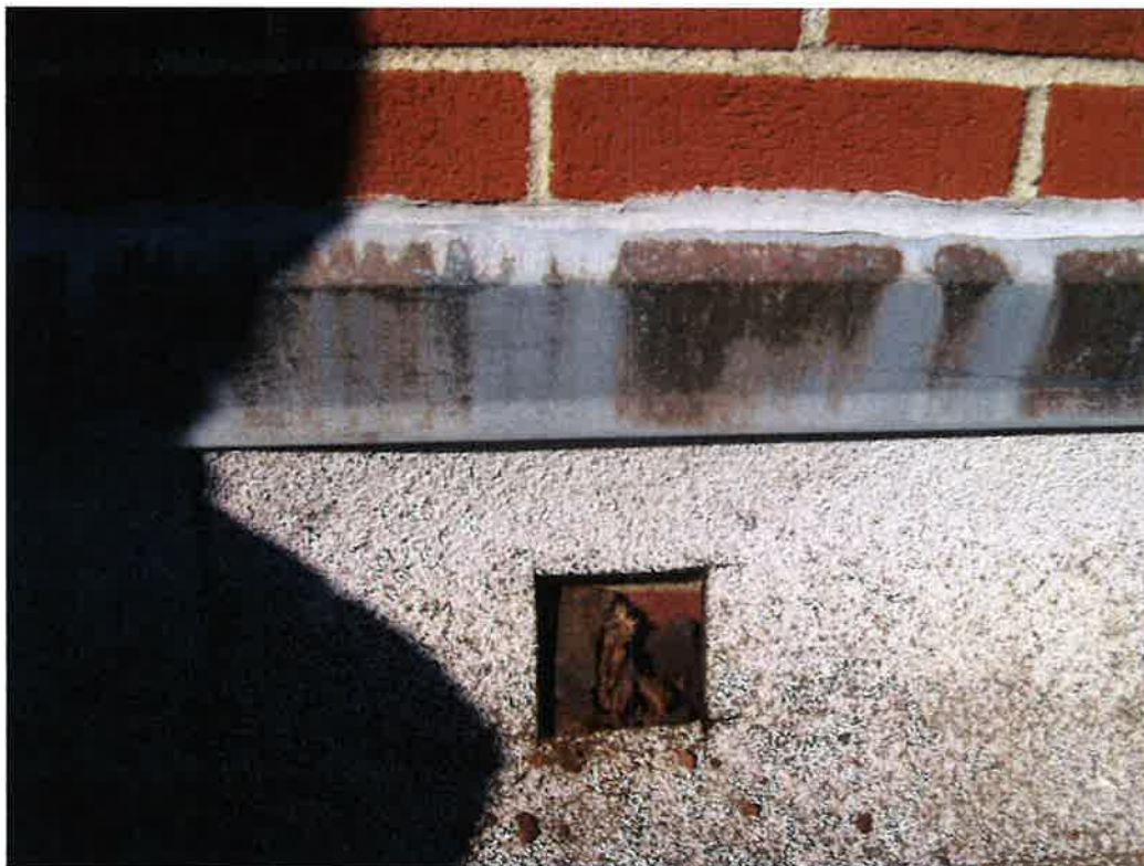
1953 and 1991 Wall junction-cold application, fiberboard, brick wall
