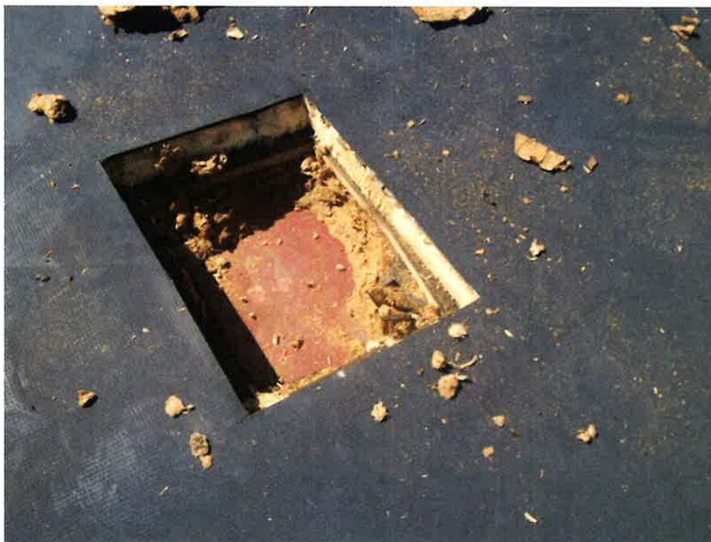
1953 Built up roofing layers and exposed deck
