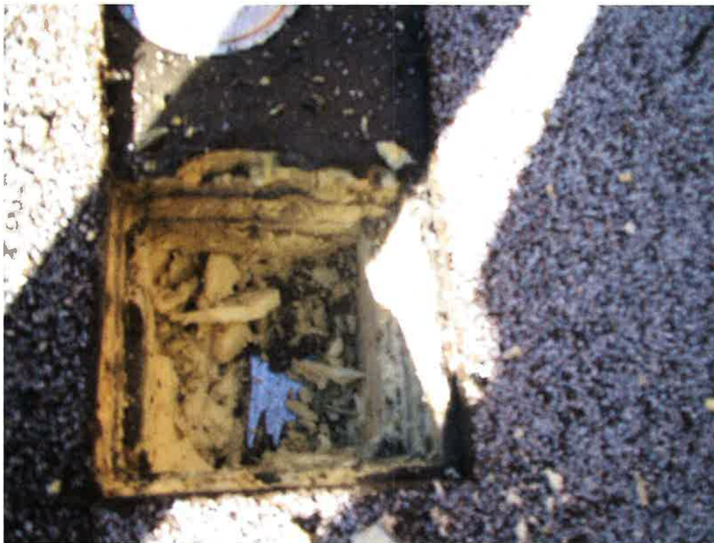
1991 Addition, low roof-built up roof layers-left side
