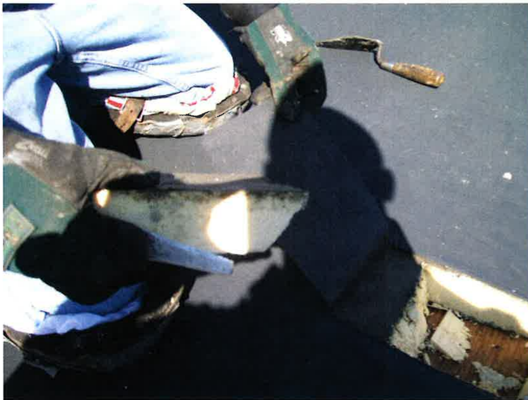
1953 Built up roof-wood deck exposed, "Poly iso" is in hand
