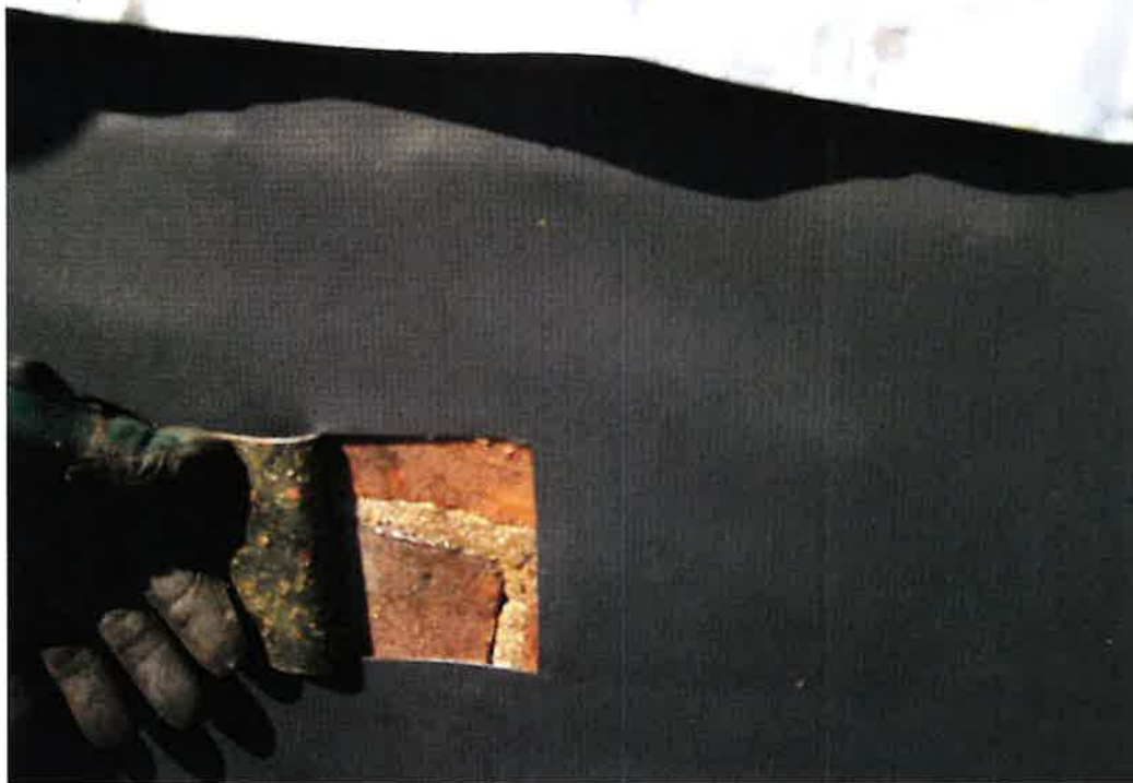
Exposed brick behind rubber membrane on gym parapet wall
