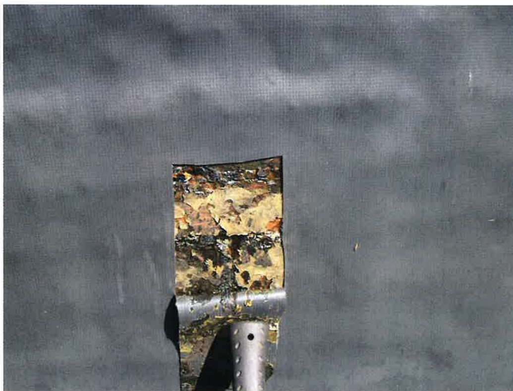
1953 Parapet wall-exposed brick and adhesive behind membrane
