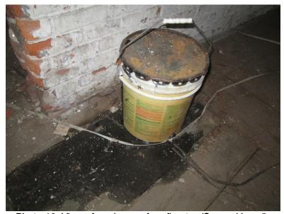
Photo 10: View of a release of roofing tar (Second Level).
