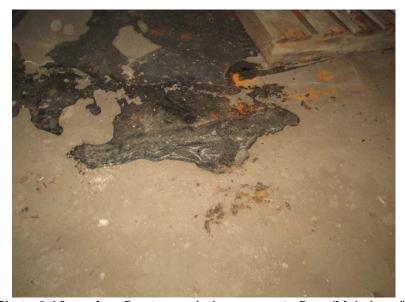
Photo 6: View of roofing tar pooled on concrete floor (Main Level).
