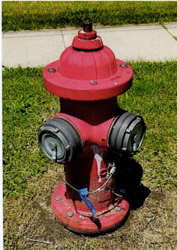
Current Storz fitting Caps on Fire Hydrant Behind Fire Station
