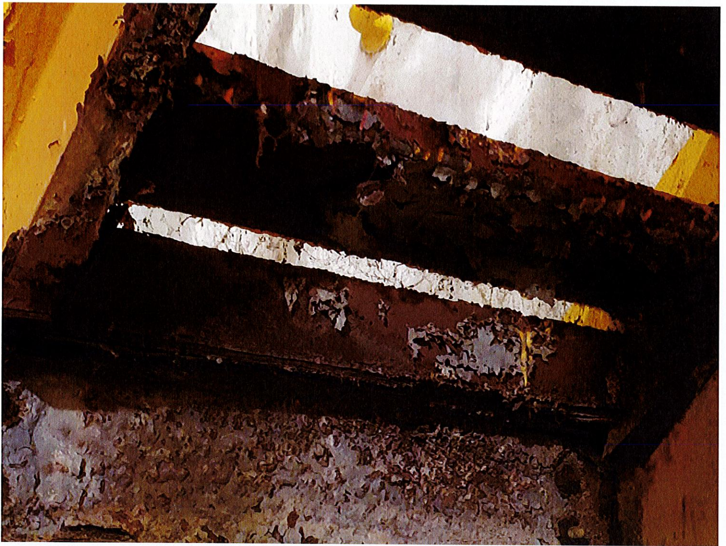
Underside of Stair Well – Corrosion has caused stairs to fail beyond repair
