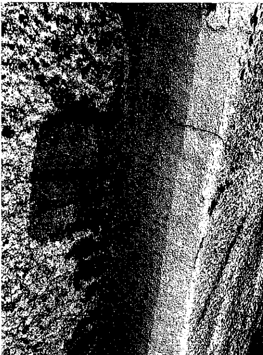
Figure 11: Spall Adjacent to Ladder
