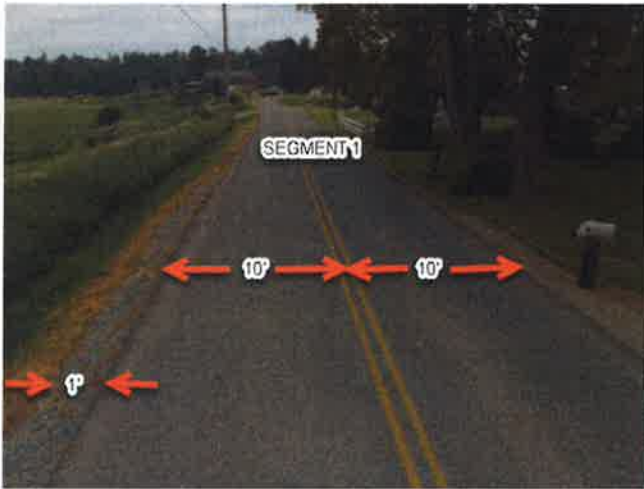
TYPICAL CROSS SECTION SEGMENT 1
