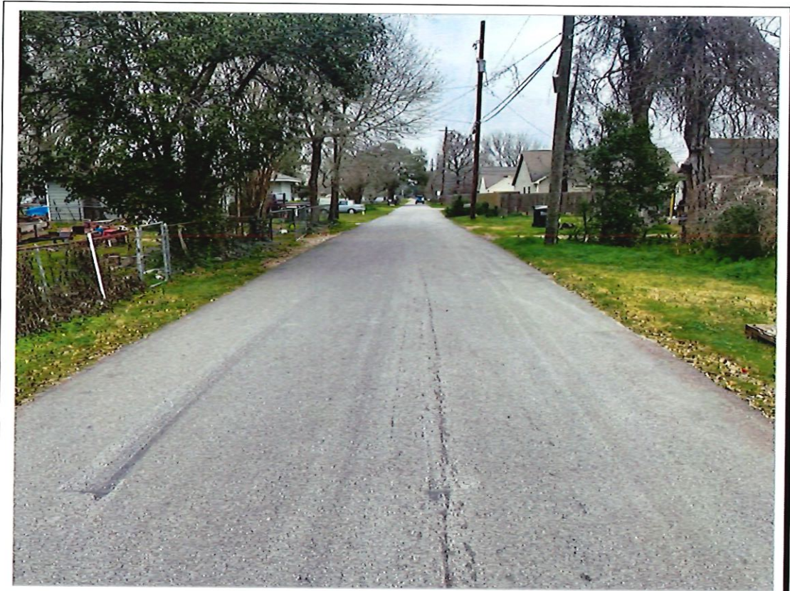
Figure 1 Anderson Street–Rehabilitated in 2024
