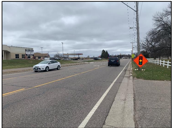
Looking south on Pine Cone Road North
