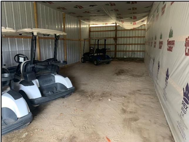
Outbuilding B - Interior
