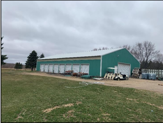
Outbuilding B - Exterior
