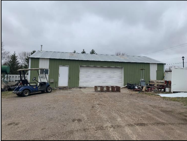
Outbuilding A - Exterior
