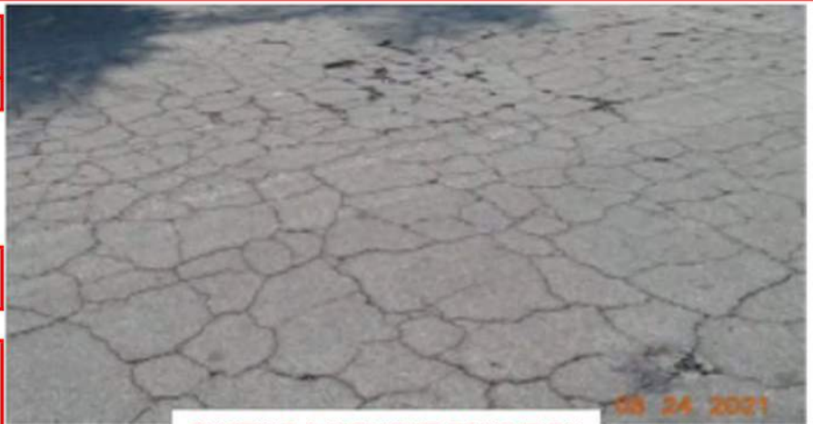
EXISTING PAVEMENT CONDITION
