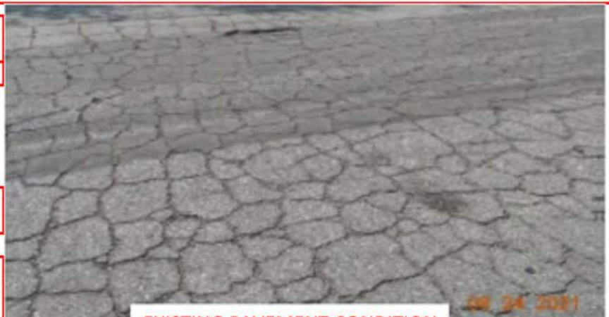
EXISTING PAVEMENT CONDITION
