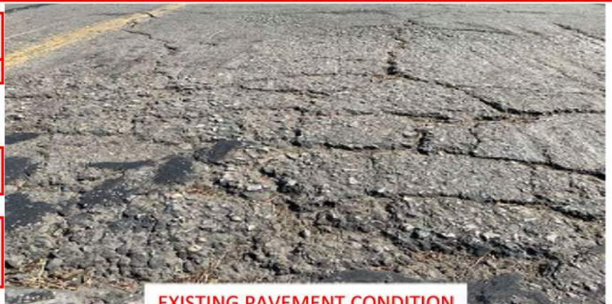
EXISTING PAVEMENT CONDITION
