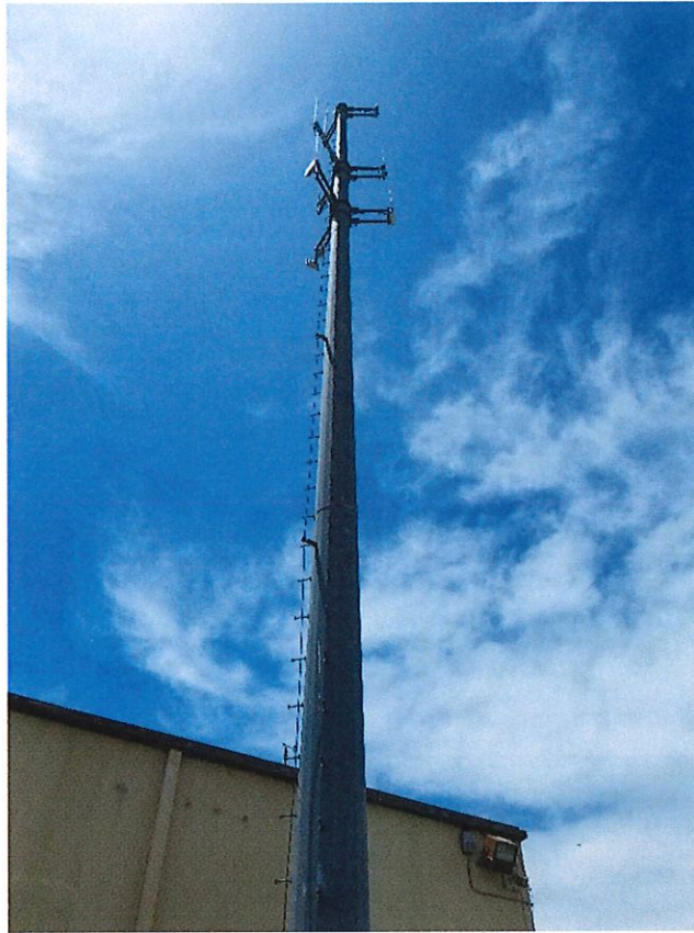
Existing Pole – 30' Deep Concrete Base
