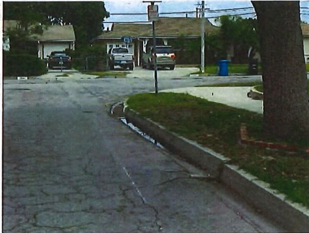
Figure 3 - Curb and Gutter Uplift
