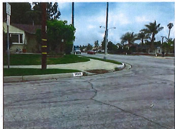
Figure 4 - Non-Compliant Ramp
