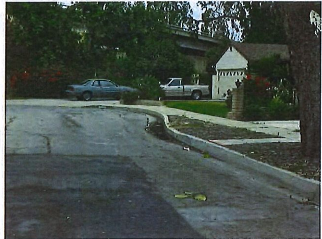
Figure 2 - Localized Gutter Depression
