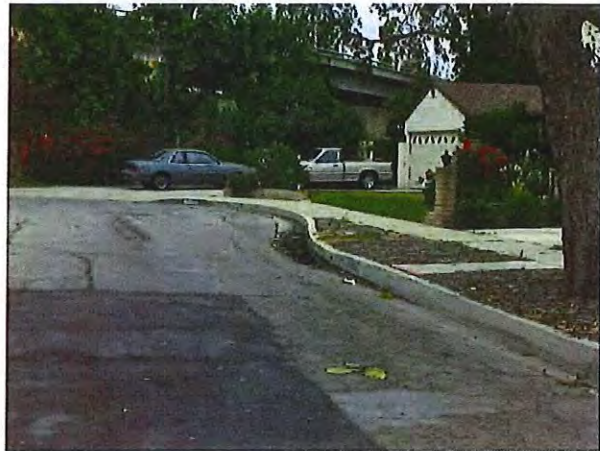
Figure 2 - Localized Gutter Depression
