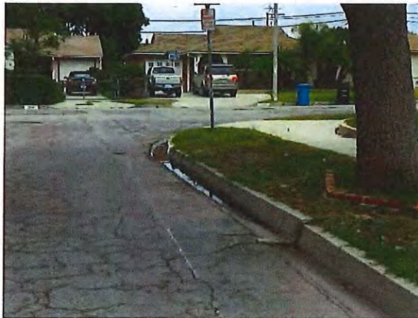
Figure 3 - Curb and Gutter Uplift
