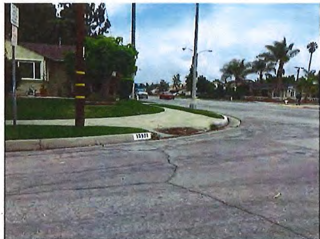
Figure 4 - Non-Compliant Ramp
