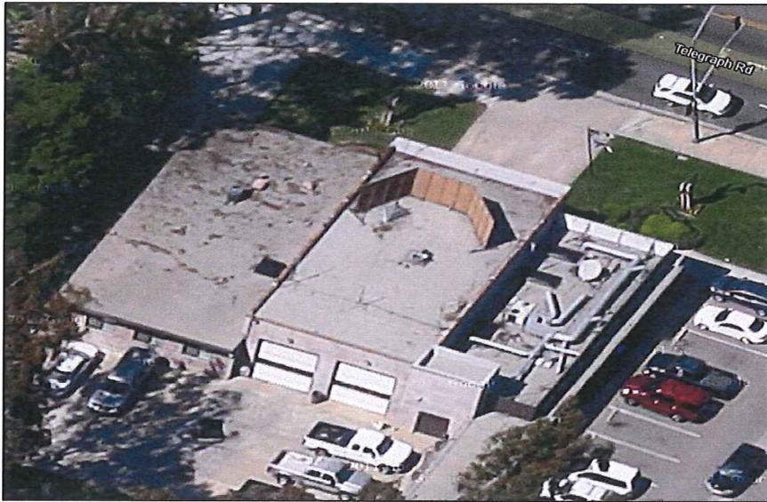
Description: Remove existing built up roof (approx 5,700 SF), install new flashings and accessories associated with new single ply roof.
