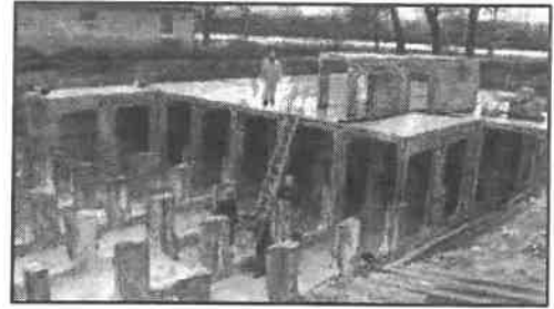
Concrete subsurface storm water detention and infiltration system
