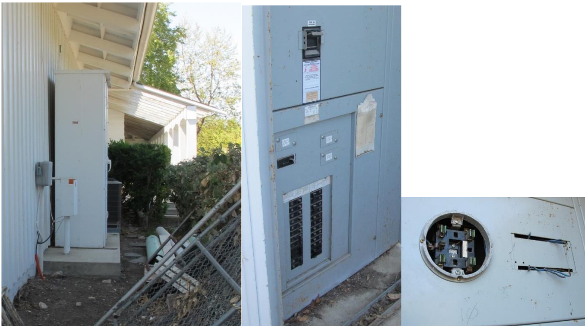
Switchboard behind Association building, interior breakers, abandoned meter socket
