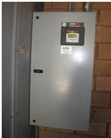
Existing ATS on back interior wall of structure
