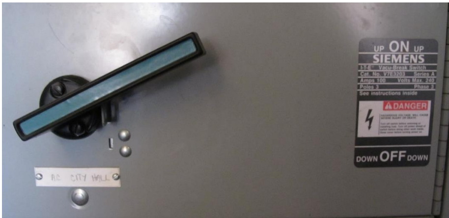
“AC City Hall” breaker in main switchboard
