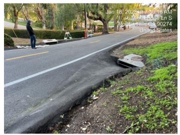
Photo 1 - Upstream 18"CMP at STA 8+17 (right side of photo) Photo 2 - (2) Sink holes were within 16 LF n/o catch basin at upstream 24"CMP at STA 7+84 (left side of photo).
