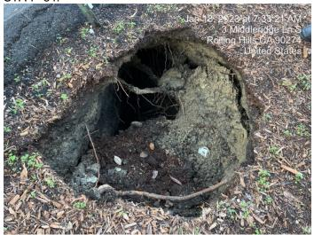
Photo 4 - Closest sink hole to catch basin was about 3' in diameter and about 8' deep (bottom of SD)
