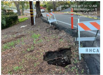
Photo 3 - Sink holes were outside of the roadway and behind AC rolled curb.
