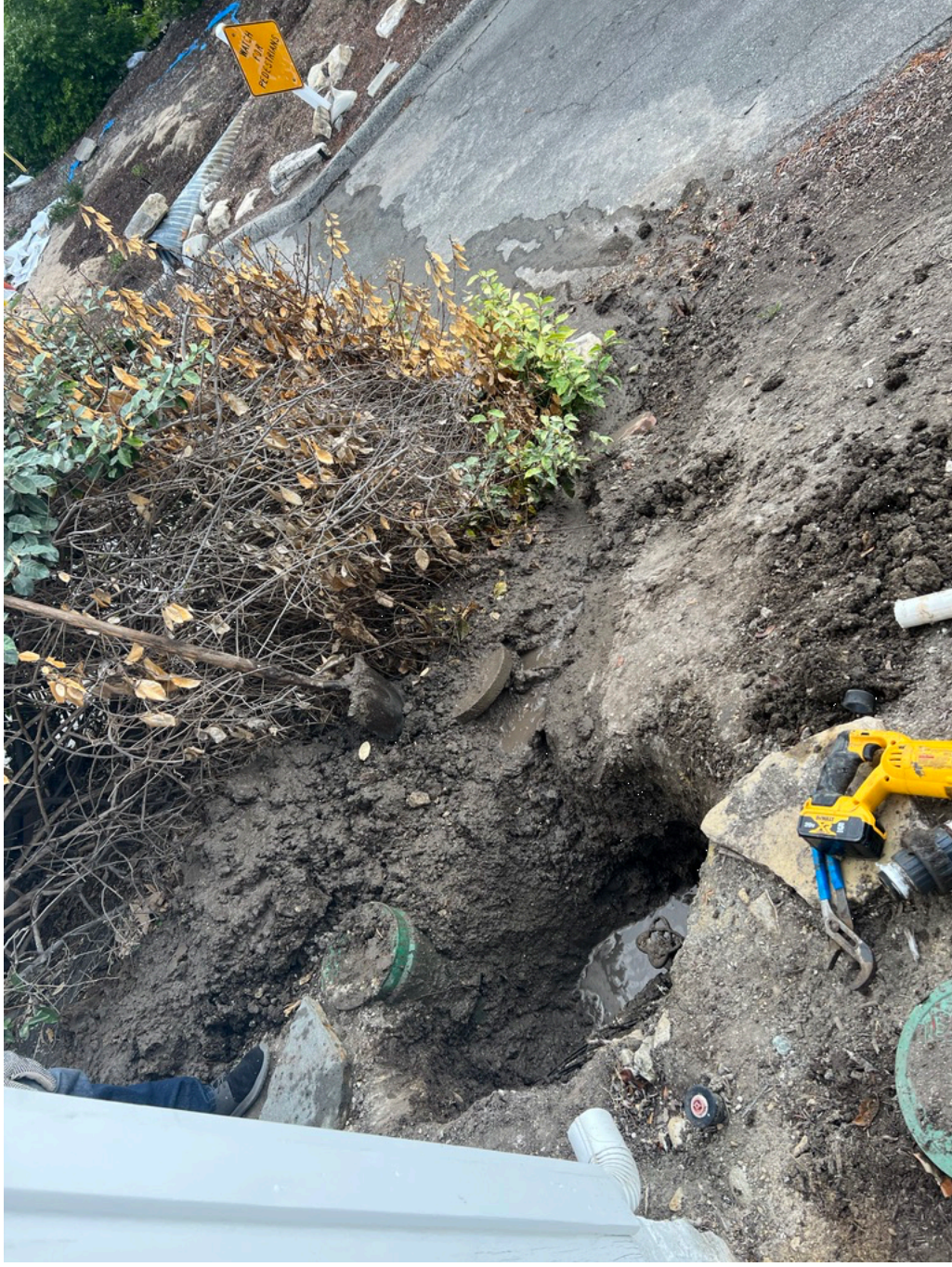
BROKEN WATER MAIN NEAR C#2 ALSO DOWN SPOUT INTO PLANTER W/ EROSION ONTO DRIVEWAY
