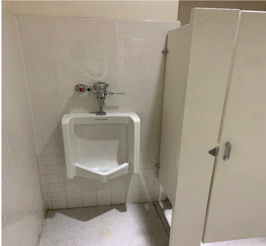
(above) Lead-containing restroom ceramic wall tile.
