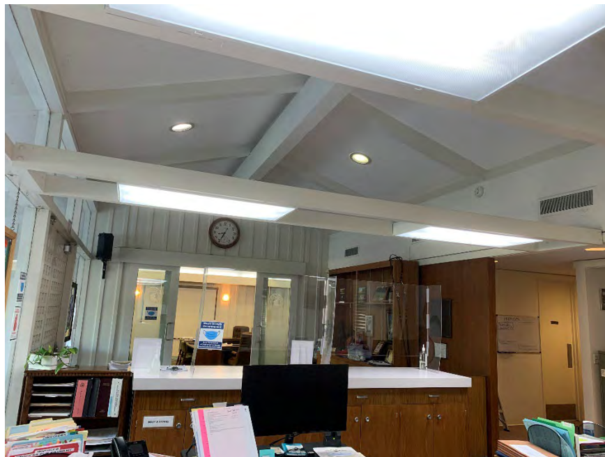
(above) Lead-based interior white trim paint.
