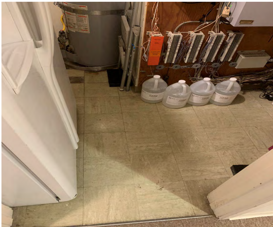
(above) Asbestos-containing 9" floor tile/mastic.
