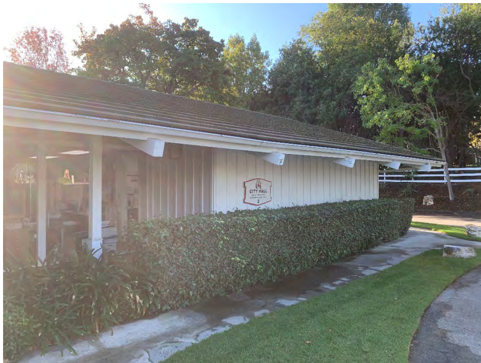
(above) Trace-asbestos containing exterior stucco overhang.
