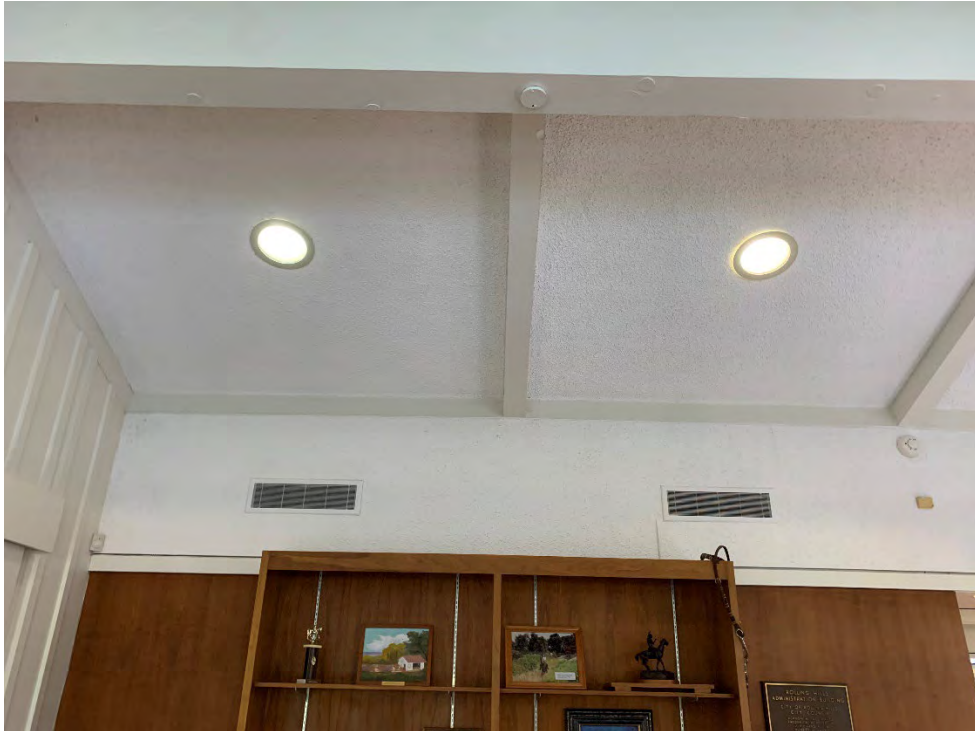
(above) Asbestos-containing acoustic ceiling and ceiling plaster.
