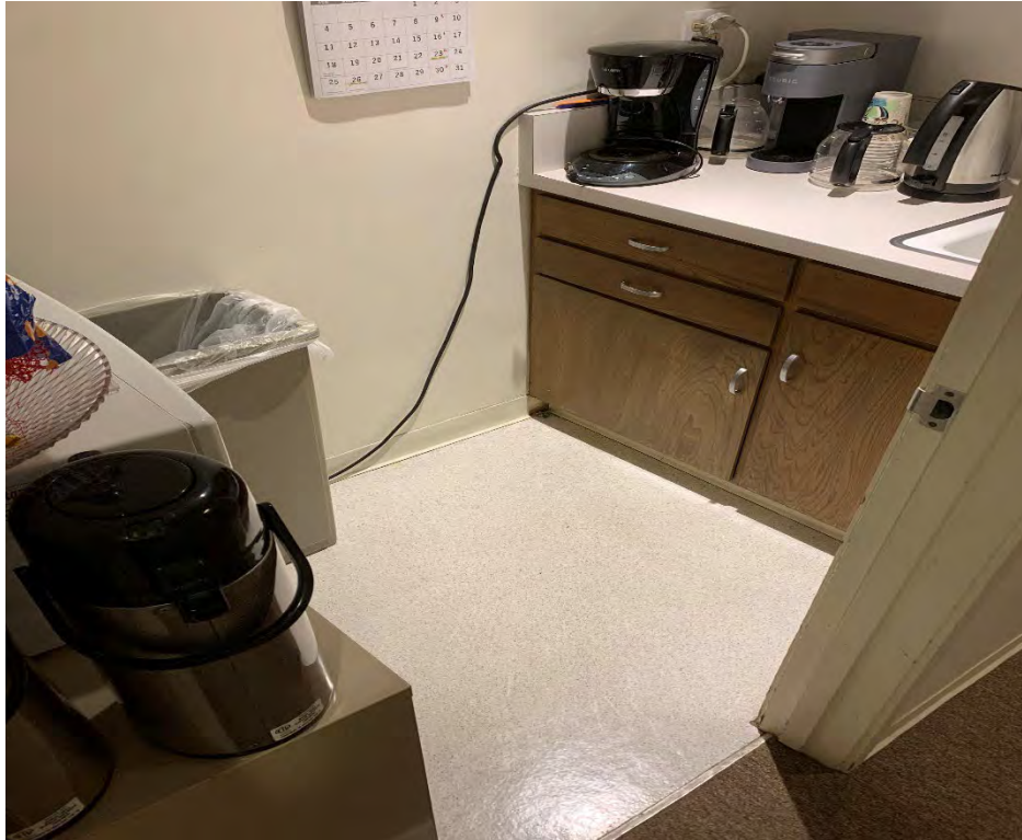
(above) Asbestos-containing linoleum (multi-layered).
