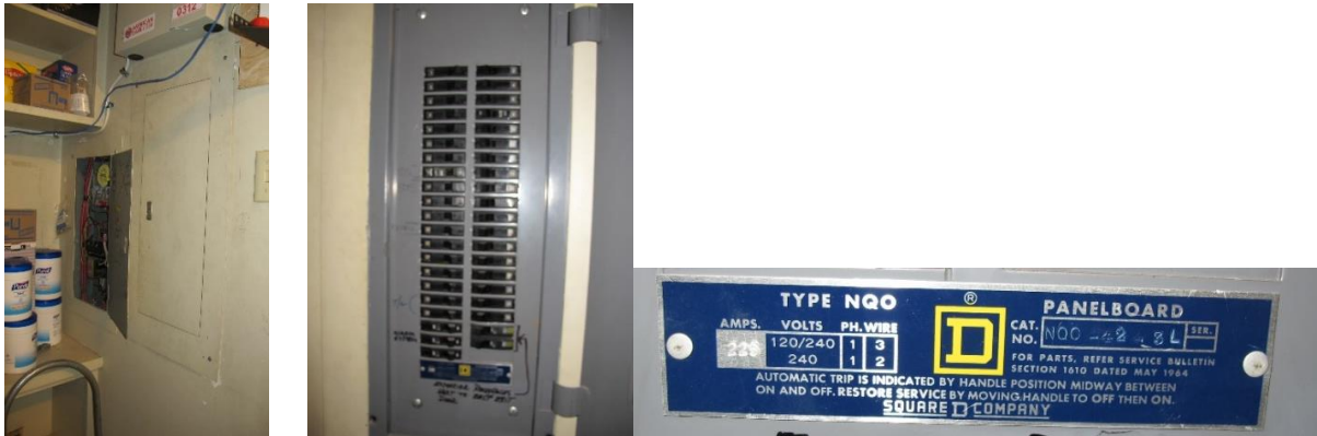
Existing City Hall branch panel exterior, interior, and nameplate
