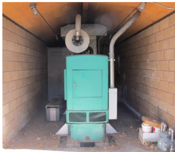
Inside of structure viewing existing generator with switchboard and ATS behind (ATS not visible in photo)
