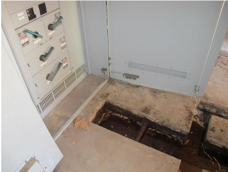
Main switchboard with doors open, branch breakers, fuel moat, and insufficient working clearance
