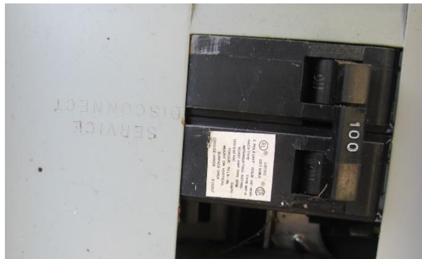
Existing panel and breaker labeled "service disconnect" at back exterior of City Hall building
