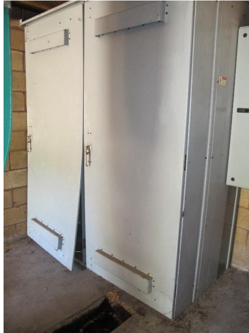
Existing main switchboard enclosure with bent door located behind generator
