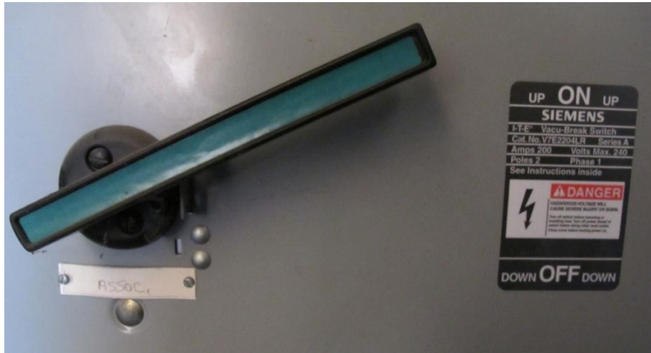
"Assoc." breaker in main switchboard
