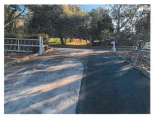
The minimum sight distance for this type of roadway shall be 155-feet for a 25-mph speed limit. The existing driveway meets and exceed the minimum sight distance requirement, furthermore the widening of the existing driveway aisle is a significant improvement and will provide better access in and out of the property. However, the lack of termination to the existing improvement within the easement poses safety concerns for
