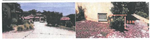
FIGURE 9 OVERALL, LOT XXX MAKES USE OF EXTENSIVE HARDSCAPING IN AND AROUND STRUCTURES. DUE TO HOME CONSTRUCTION THAT INCLUDES STUCCO WITHOUT WEEP SCREENING, THERE IS NO NEED FOR A NON-COMBUSTIBLE ZONE. HOWEVER, ALL MULCH WILL NEED TO BE REMOVED WITHIN 5 FEET OF FOUNDATION VENTS.
