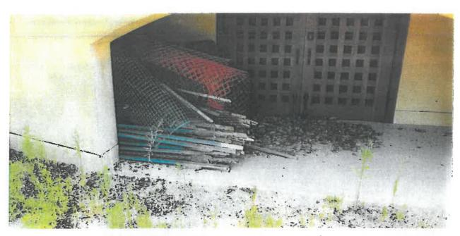
FIGURE 11 BECAUSE IT IS AN EMBER TRAP (AS EVIDENCED BY CURRENT LEAF BUILD-UP), CLEAR AWAY COMBUSTIBLE MATERIAL FROM COVERED STORAGE ENTRY.
