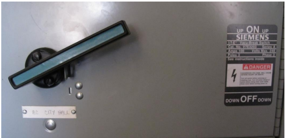
“AC City Hall” breaker in main switchboard
