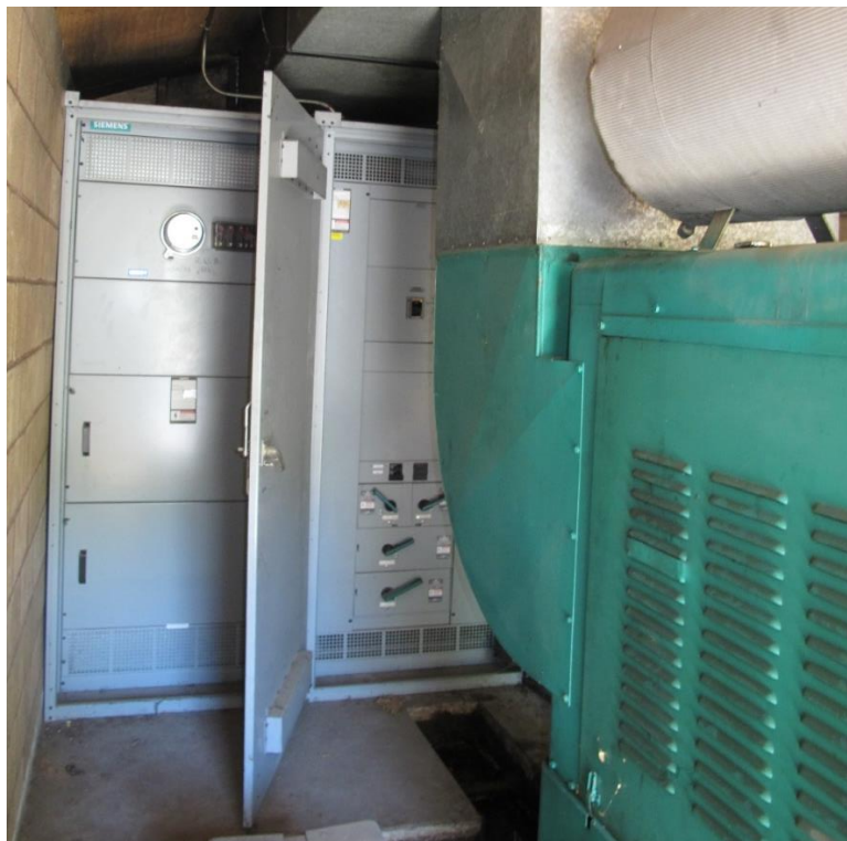
Main switchboard with doors open, SCE meter, main and branch breakers, and fuel moat
