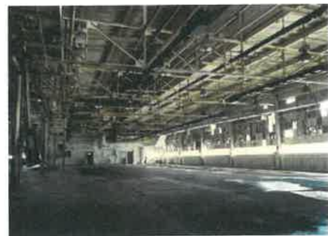
Figure 4: Interior of the Ford Valve Plant, showing the original steel frame and concrete floor
