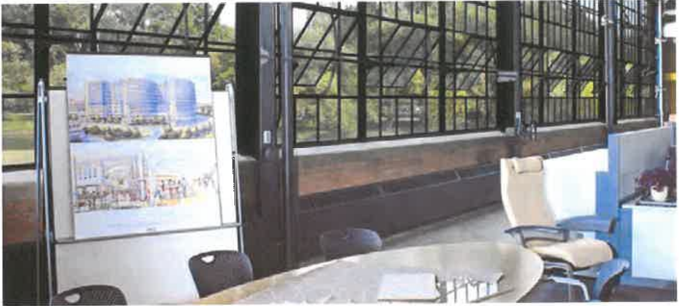
Figure 7: The Zedler office renovation can be seen in the window restoration. Rick Cox developed a method to install energy-efficient windows in the original frames. Over 9,000 windows were replaced into the original steel frames, which had been stripped and repaired.
