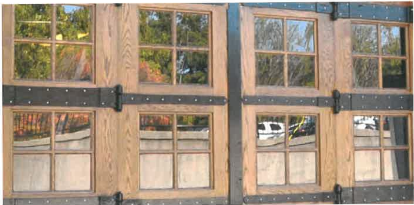
Figure 8: The window frame on the third floor of the Henry Project. The original window frame was removed and replaced with a new one made of heavy-duty steel and wood.
