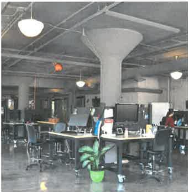
Figure 12. While a lot of the interior has been modernized for use as open industrial loft style office space, the original flared "mushroom" columns designed by Albert Cox remain. The unique, load-bearing design of these columns allowed for maximum support in minimal space. The columns are built of fireproof reinforced concrete. Evolutionary design in the 1950s.
