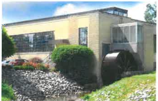
Figure 6: In 1998, the decision was made to rebuild the disintegrating water wheel. Plymouth-based Castle Enterprises reassembled and re-bolted the wheel using the same specifications as the original. The fabricating firm was able to follow the rediscovered plans from a similar water wheel at one of Henry Ford's other early factories. Two sets of bearings were produced to allow a spare set for future replacements. The final phase included installing custom buckets commissioned by the Coxes. In 2017, at the Coxes' expense, the wheel was again redesigned and rebuilt for the community enjoyment. This time, the wheel was redesigned by Mr. Cox using stainless steel. The engineering analysis indicated that this new wheel could last close to 100 years, honoring and celebrating the ingenuity of the water wheel in Northville.
