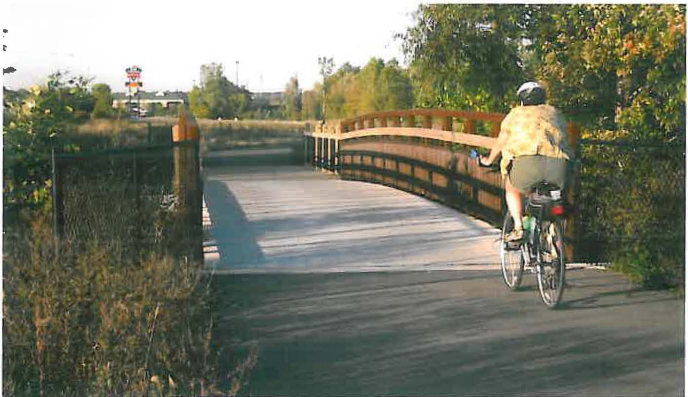
Trail bridge over Mill Creek for multi-use linear park was constructed utilizing sheet pile abutments which minimized construction impact on the Creek.
