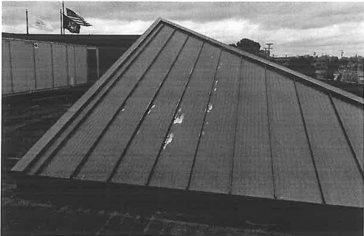
Photograph 2 – View showing range in size of delamination.
