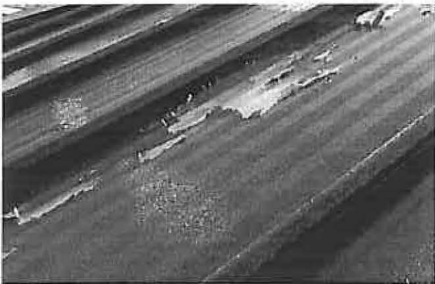
Photo 6 - DELAMINATED PAINT
