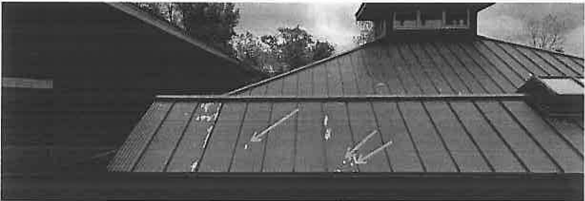
Photograph 6 – Test performed on panel with no exhibited delamination, then two tests performed on panel with significant delamination.
