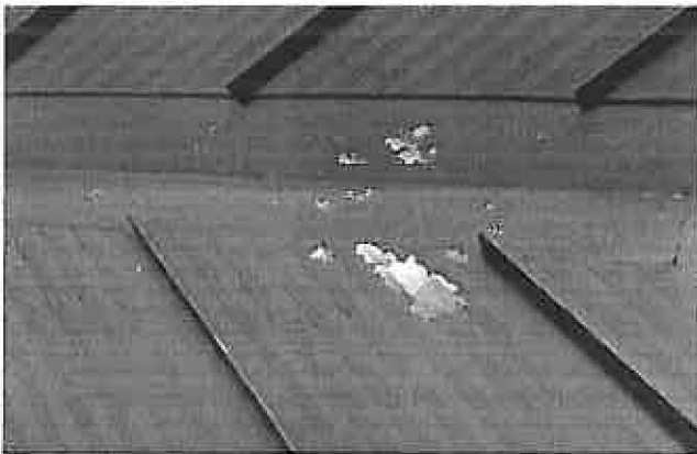
Photo 10 - DELAMINATED PAINT ON VALLEY SHEET METAL AND ADJACENT ROOF PANEL
