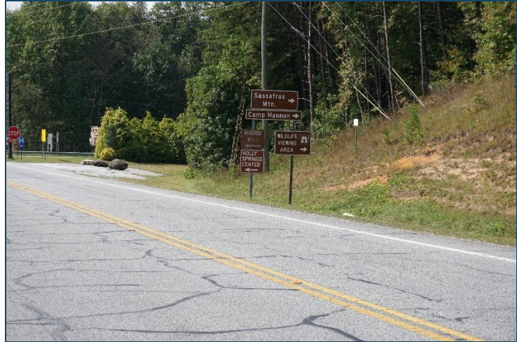
An example of steep slopes along Highway 11.
