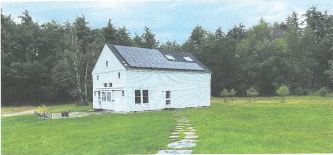
Above photo: Accessory dwelling to be demolished (photo taken facing north/northeast);
