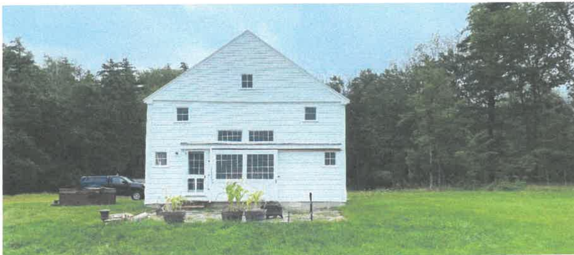
Below photo: West façade of accessory dwelling to be demolished (photo taken facing east).
