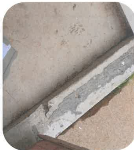
Chicken Coop Threshold - Dam Proofing
