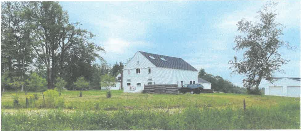
Above photo: Accessory dwelling to be demolished (photo taken facing southwest);
