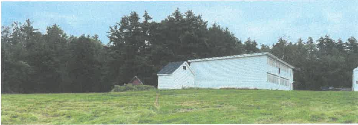
Above photo: Chicken barn and detached well house, which will be removed (photo taken facing east);
