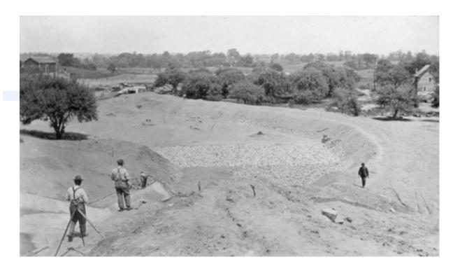
Enlarging the Erie Canal into the 1000 Ton Barge Canal required the engineers and surveyors planning the work to have portions of the canal drained as the work progressed westward. Surveyors and workers are shown here west of Spencerport looking over a newly drained and filled stretch of the canal.
