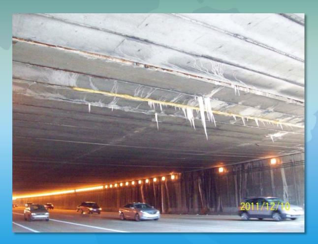
Leaking under structure has caused hazardous conditions on I-696.
