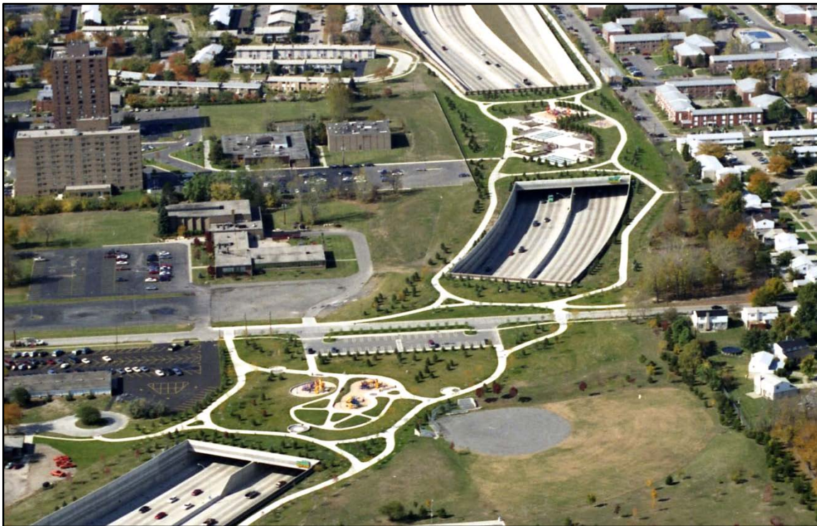
Bridge Decks over I-696
