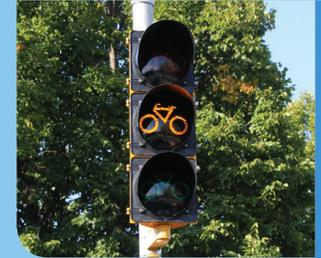
**Bicycle signal heads** are used in conjunction with existing traffic signals to indicate bicycle-specific timing sequences.
