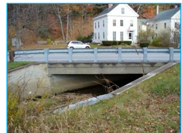
Main Street Bridge
