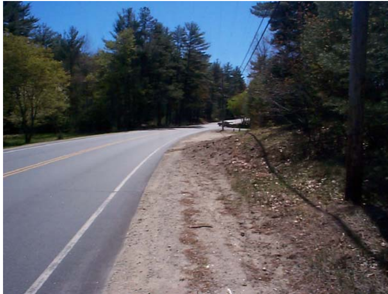
Looking east at the NH 130-Bohannon Bridge Road intersection
