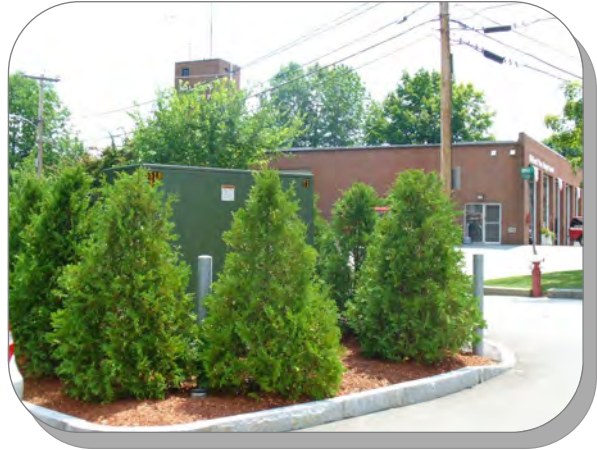
Shrubbery conceals this electrical equipment while allowing easy access for repairs.
