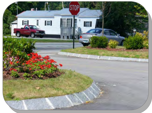
Curb cuts are well defined with granite blocks.
