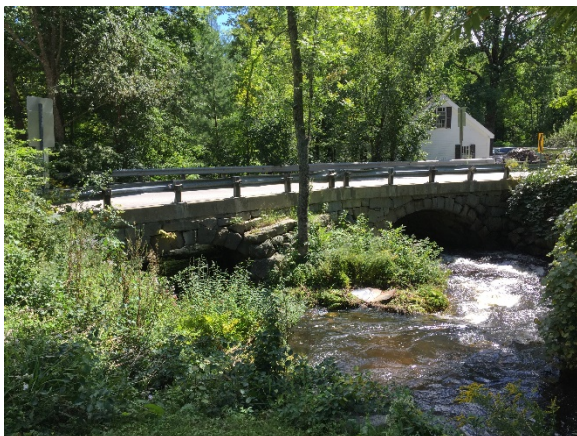
West Wilton Bridge Image Credit: Wilton Planning Board & NRPC
