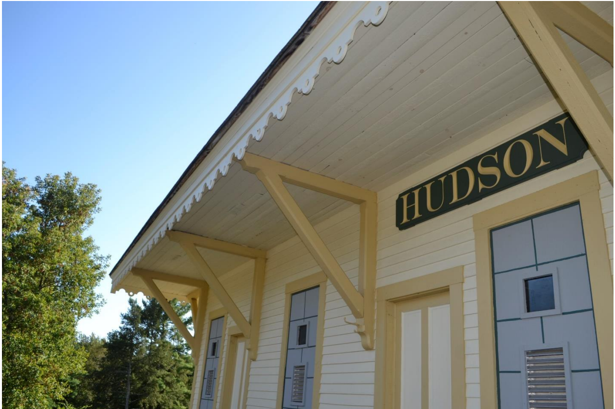
Benson's B&M Railroad Depot
