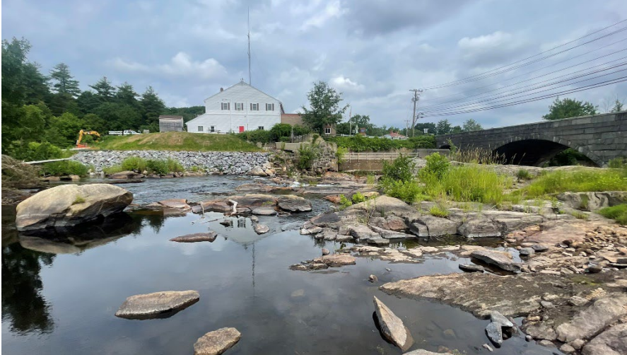
Figure 4. Site of the former Merrimack Village Dam, Merrimack.
