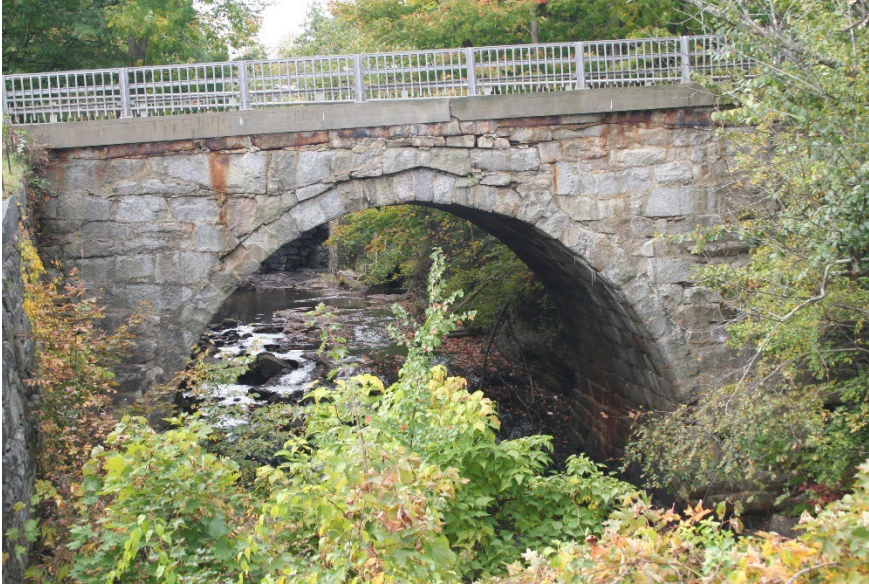
Figure 11. Mill Street Bridge, Greenville.
