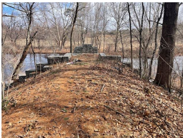
Figure 12. Bridge Abutment of the Milford-Manchester B&M Rail Bridge, Amherst.
