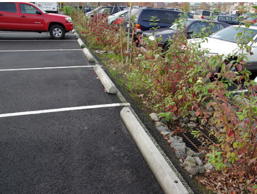
Low Impact Development (LID) strategies include stormwater bioinfiltration swales within parking lots.
