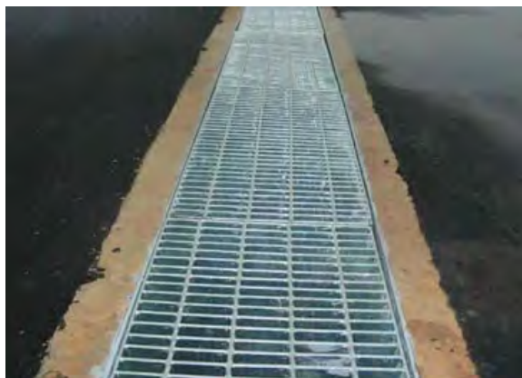
Figure 25 – Linear Drainage Grate for Collecting Sheet Flows
